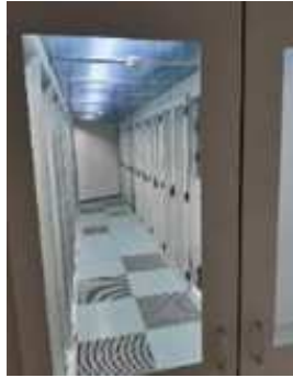
Cold aisle capping and blanking panels Left – Germany Right – UK
